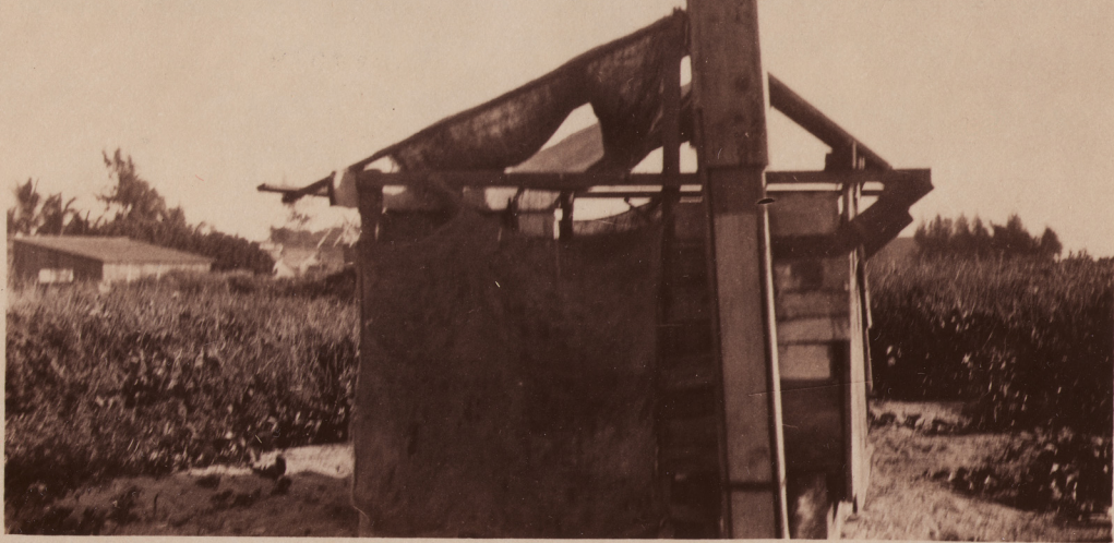
Dilapidated open privy vault Filipino Strike Camp, Kapaa, Kauai.
